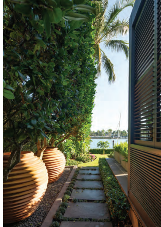
The louvered cladding meets Miami's stringent wind-load requirements, and can rotate 150 degrees and be closed via an app.
